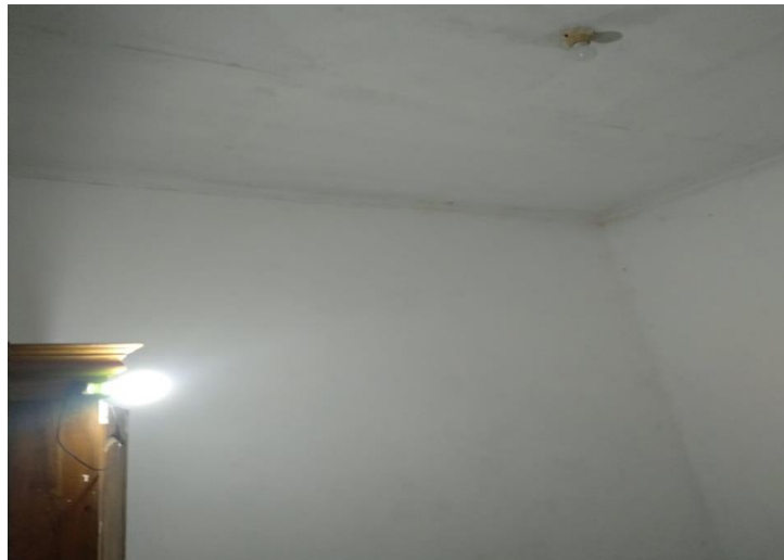
Gambar 8 Implementasi DOLAR ENERGY
